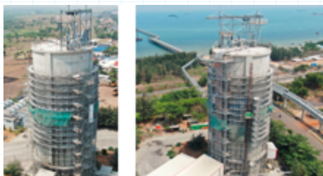
Install platform scaffolding Level 17
